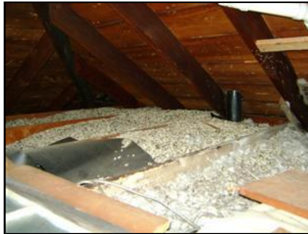
9.0 Picture 1 Vermiculite insulation in attic.
