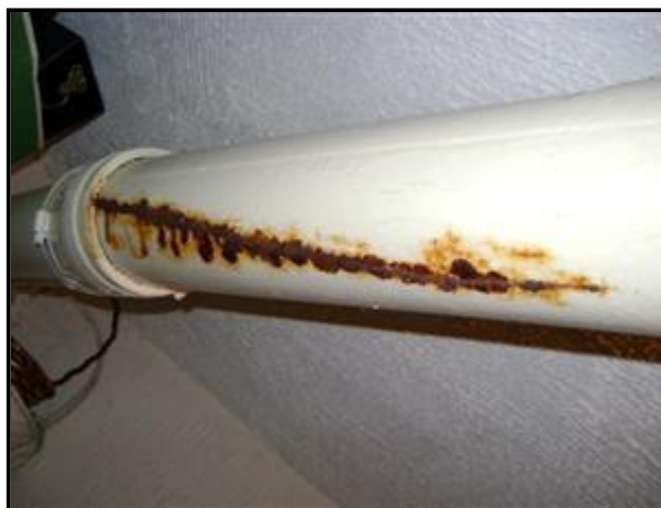
6.0 Picture 2 Cracked waste line in basement.
