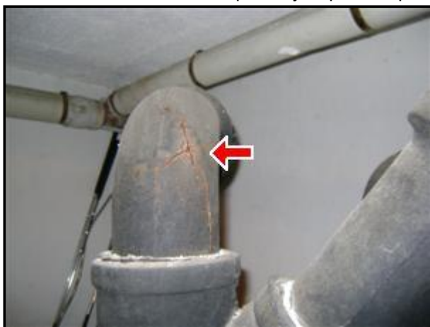
6.0 Picture 1 Cast iron waste line in basement.
